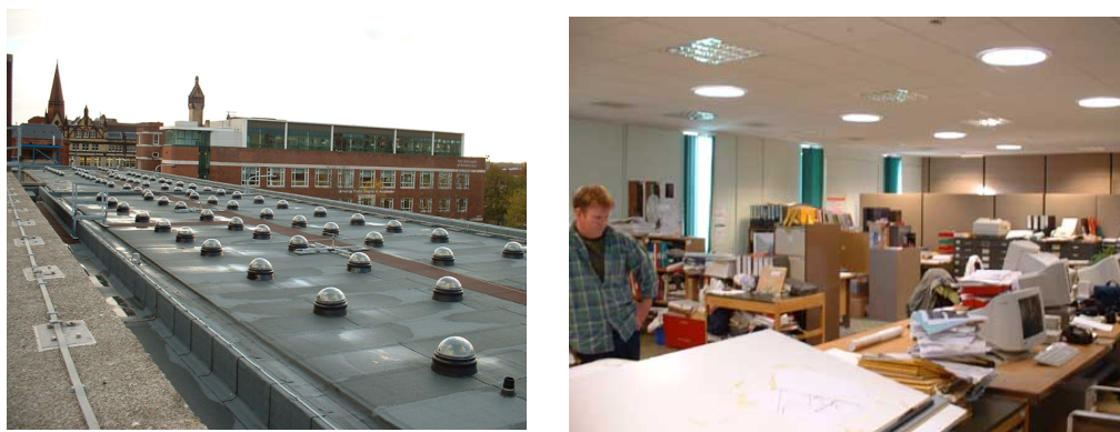
Figure 9. Internal and external view of large installation.
