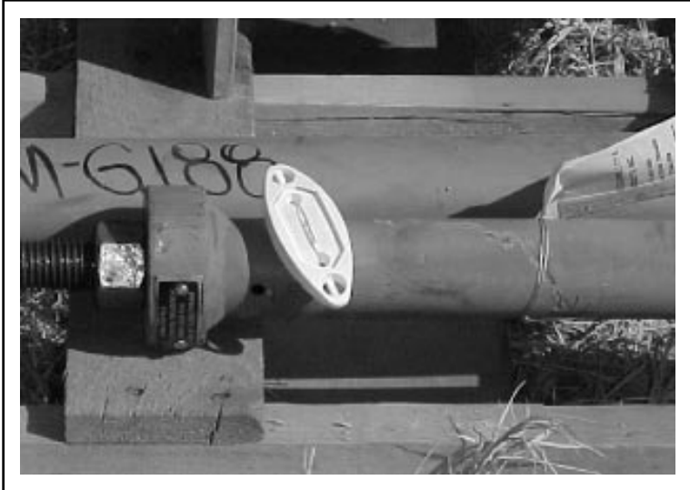
Figure 1. RFID Tag Attached to Pipe Support
