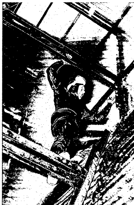
Fig. 3 Inspection of framing in plenum area of crossflow tower.
