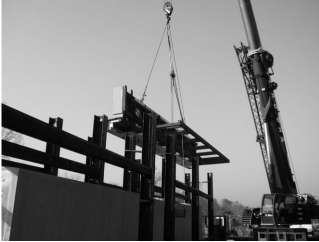
Fig. 3-9. Stone truss panel being hoisted from transportation vehicle; note the steel frame back-up behind the stone panels
