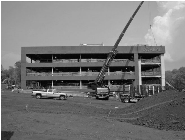
Fig. 3-8. Stone truss panel being installed
