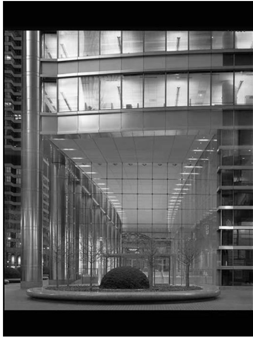
Fig. 3-25. UBS Tower, Chicago, IL
