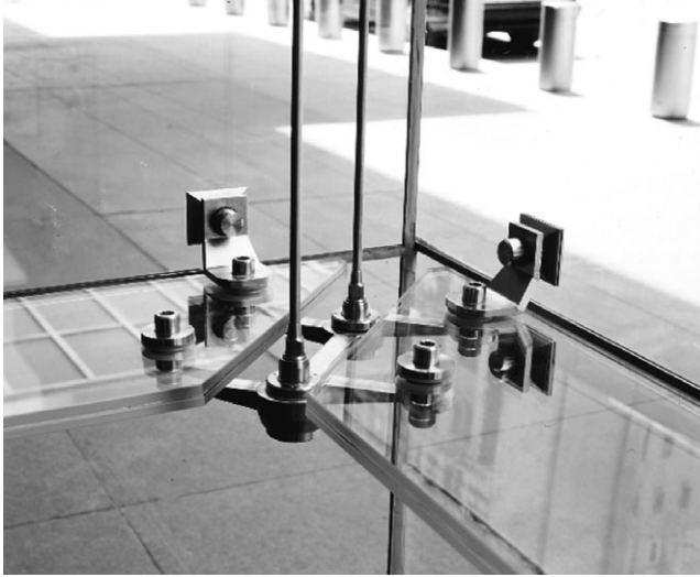
Fig. 3-23. Complex glazing connections; example of point-supported glazing Source: Courtesy of W&W Glass, LLC; reproduced with permission
