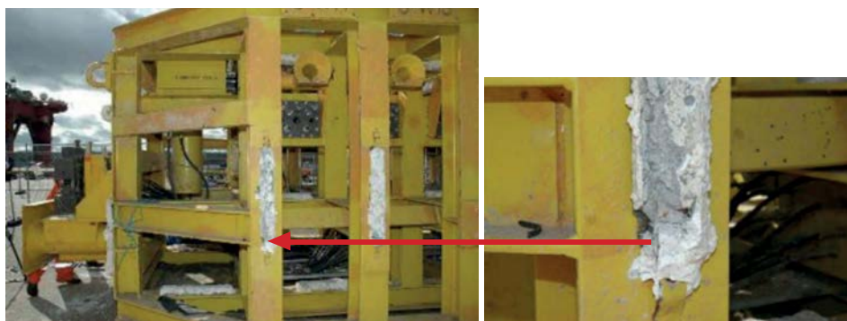
Figure 4 Subsea umbilical termination unit recovered after 10 years subsea, showing extensive wastage of the aluminium anodes but no corrosion of the steel structure
