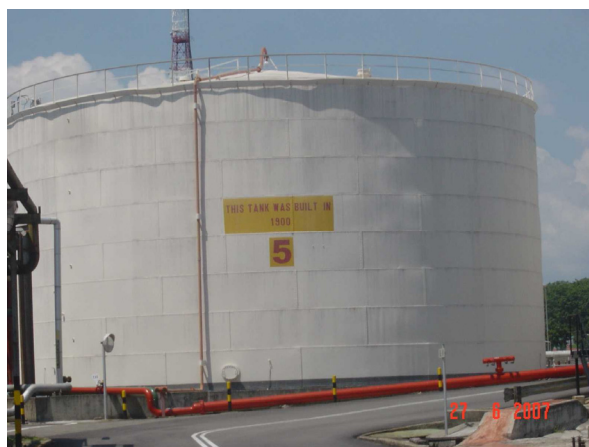
Figure 2 A tank constructed in 1900 and still in use (Asia) Courtesy of Shell
