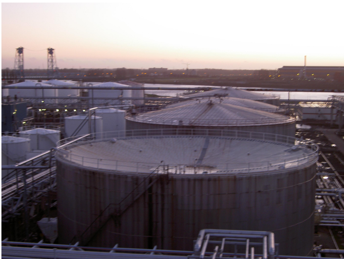
Figure 2 Roof collapse due to vacuum in the tank
