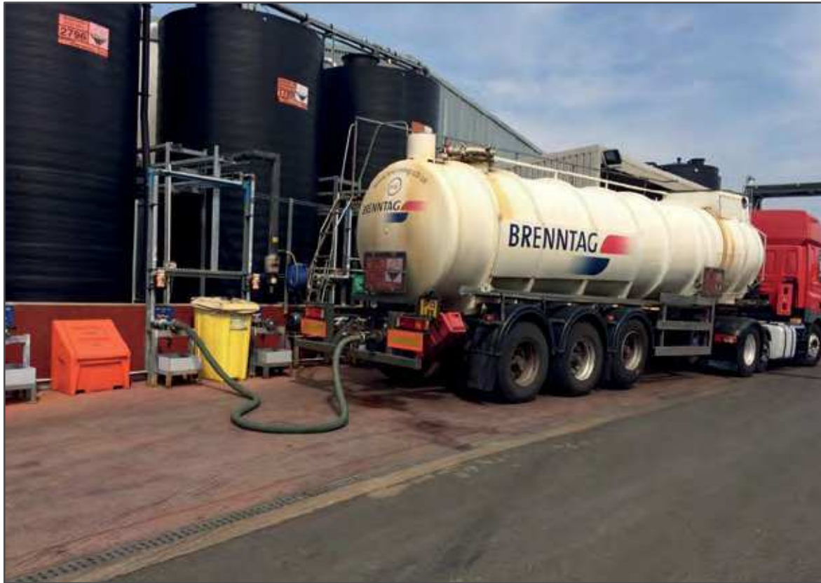
Figure 4: A tank being filled by discharge from a road tanker
