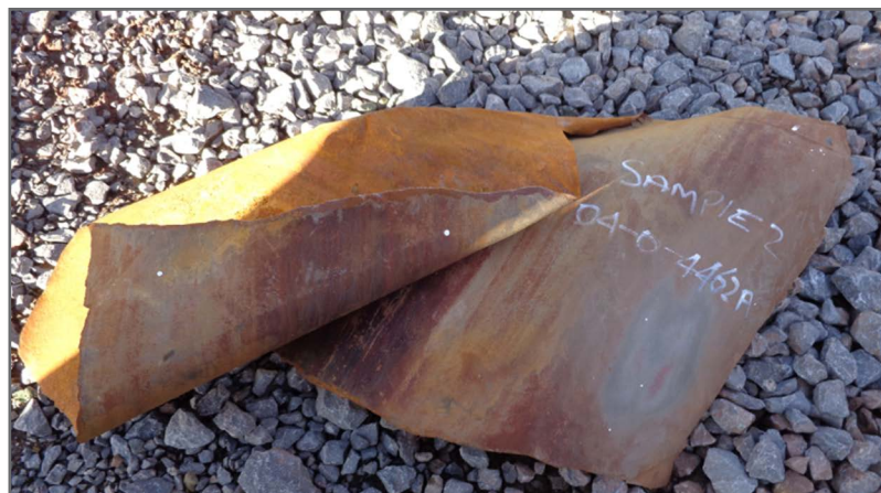
Figure 2-1 Photo showing the displaced section of line
