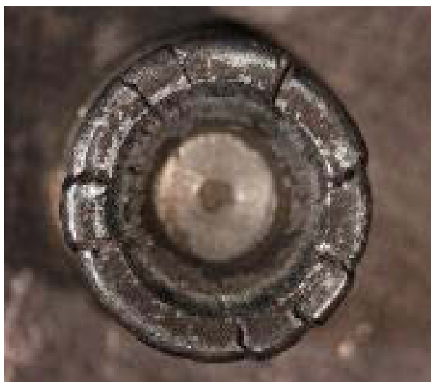
Figure 5: Split Marks/Internal Fractures Example on Die Side of Joint (Shown Riveted with PIP Die)
