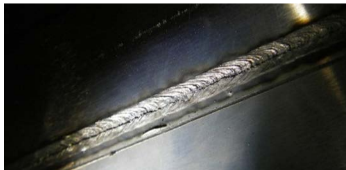
Figure 5: Surface Crack Example
