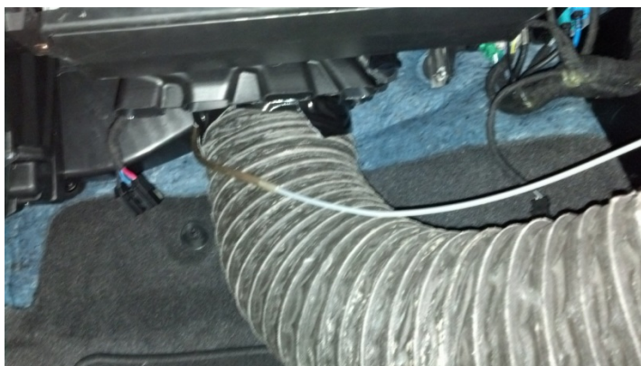
Figure 2: Particle Filter and Blower Motor Removed from HVAC, Hose Connected to Hole for Blower Motor
