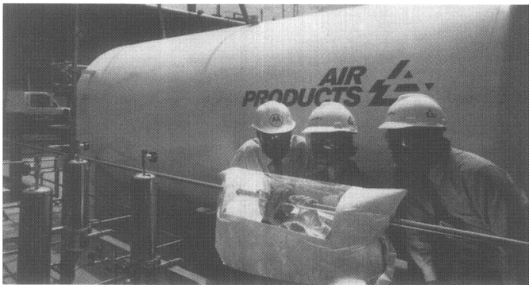
Fig. 1-7. The use of compressed gases in the manufacture of semiconductors for the electronics industry has become a major application. Here, a portable “clean room” and advanced pipe welding techniques are used to ensure highest possible gas purity.
