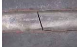
Transverse crack.
