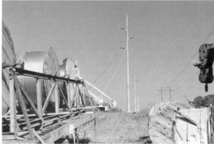
Figure 2—Conductor stringing
