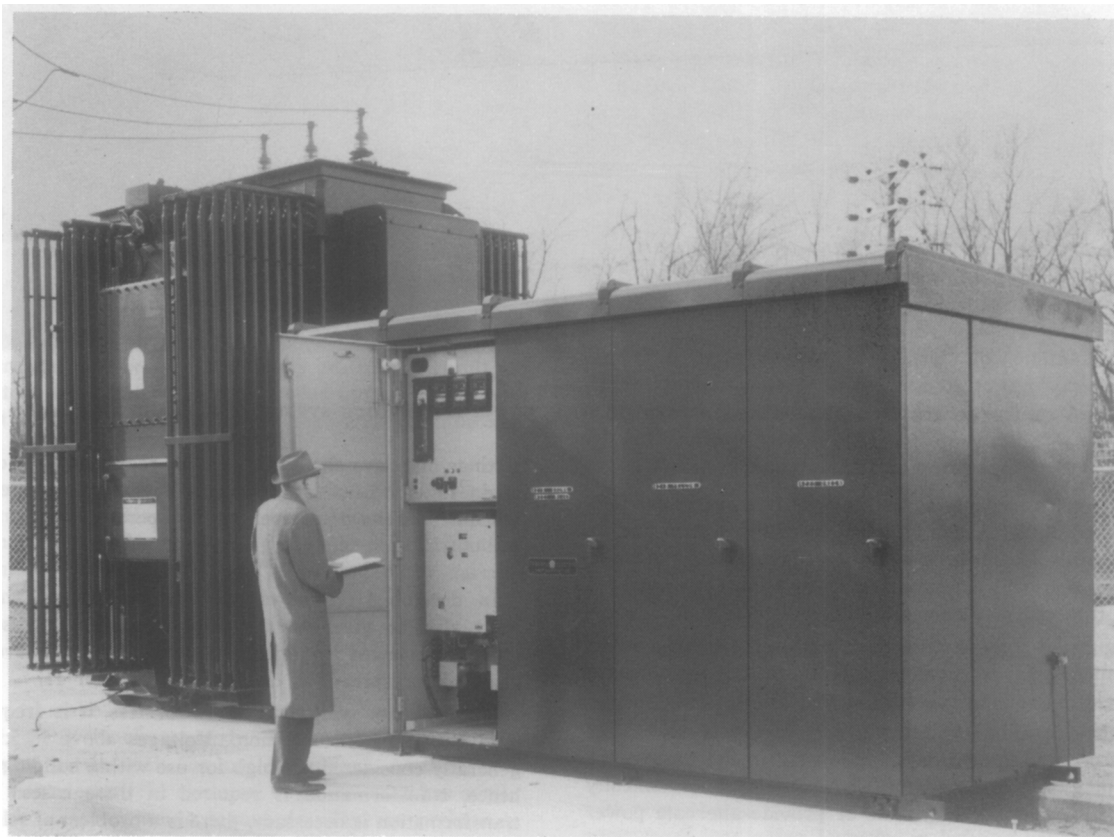
Figure 1.1 Industrial unit substation installation of 7500 kVA with load-tap-changing equipment and outdoor metal-clad switchgear
