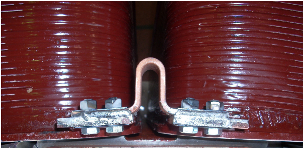
Figure 7—Solid but flexible connector shaped like an omega ( \Omega )
