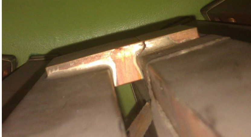
Figure 1—Pole-to-pole “T” type solid copper connector
