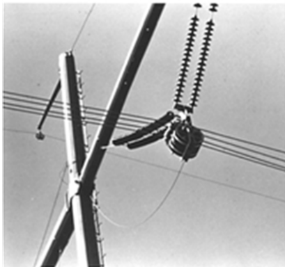
a) Application of traveler ground
