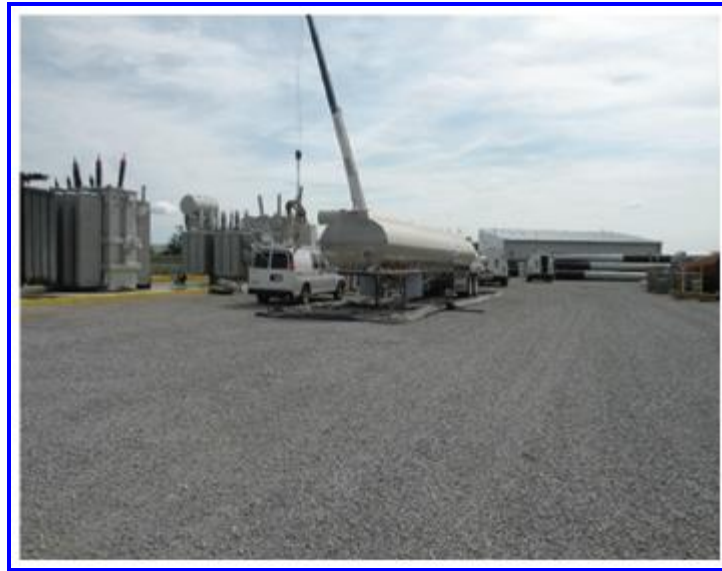
Figure 7—Containment for tanker of transformer oil in the process of filling a transformer
