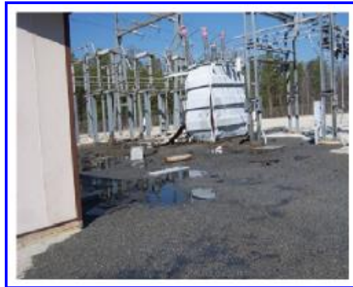
Figure 3—Ruptured transformer and resultant oil spill
