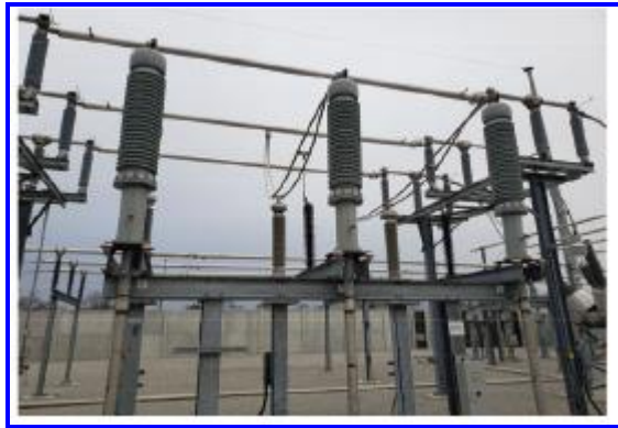
Figure 5—Cable terminations (potheads)
