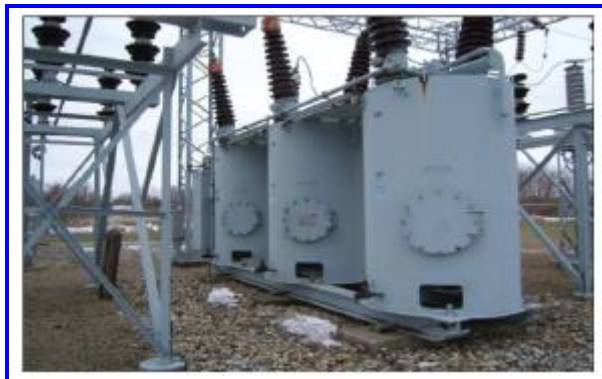
Figure 2 – 120 kV oil circuit breaker
