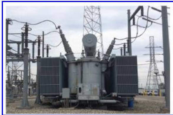
Figure 1 – Oil-filled 345 kV power transformer
