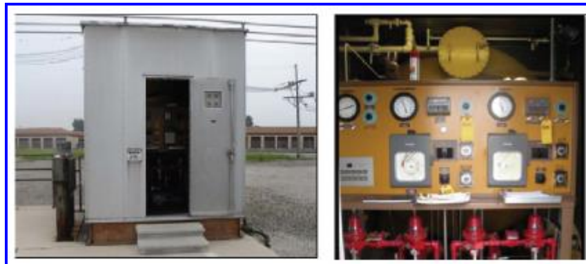
Figure 4—Oil-filled cable pumping facilities
