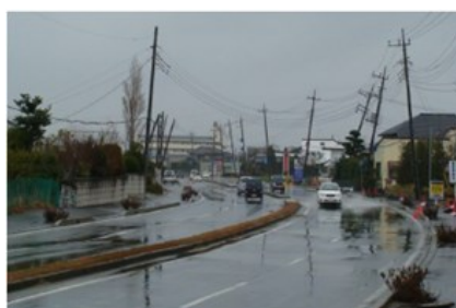
Telephone poles collapse (Hurricane)
