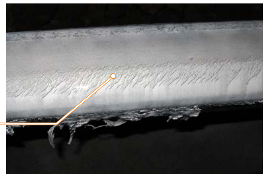
Gauge Corner Cracking (GCC)
