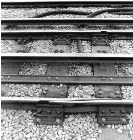
Plate 2 FB rail expansion switches
