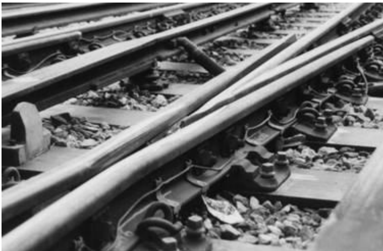
Fig. 2 Normal areas of wear on crossings
