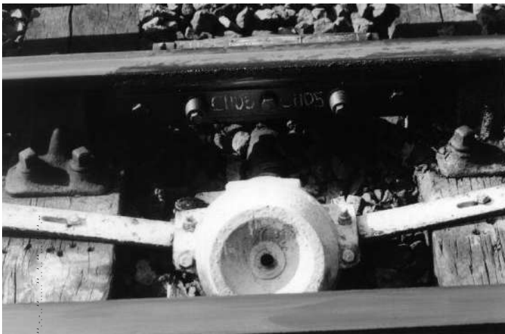
Plate 10 Portec rail lubricator
