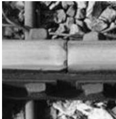
Left Plate 12 Lipped rail joint
