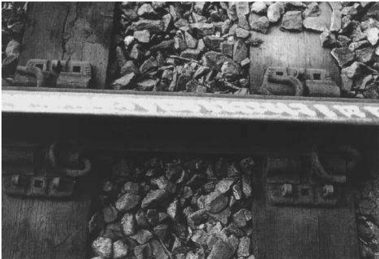
Plate 2 Rail head short wavelength corrugation. The light-coloured areas indicate high spots on the rail surface.
