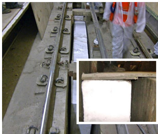
Polystyrene blocks with ply for deep pits
