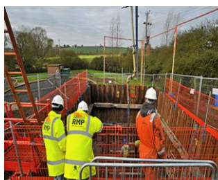
Access and edge protection system for piled trenches with hydraulic wailing
