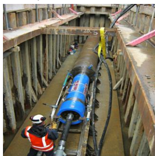
Access and edge protection system for piled trenches with hydraulic wailing
