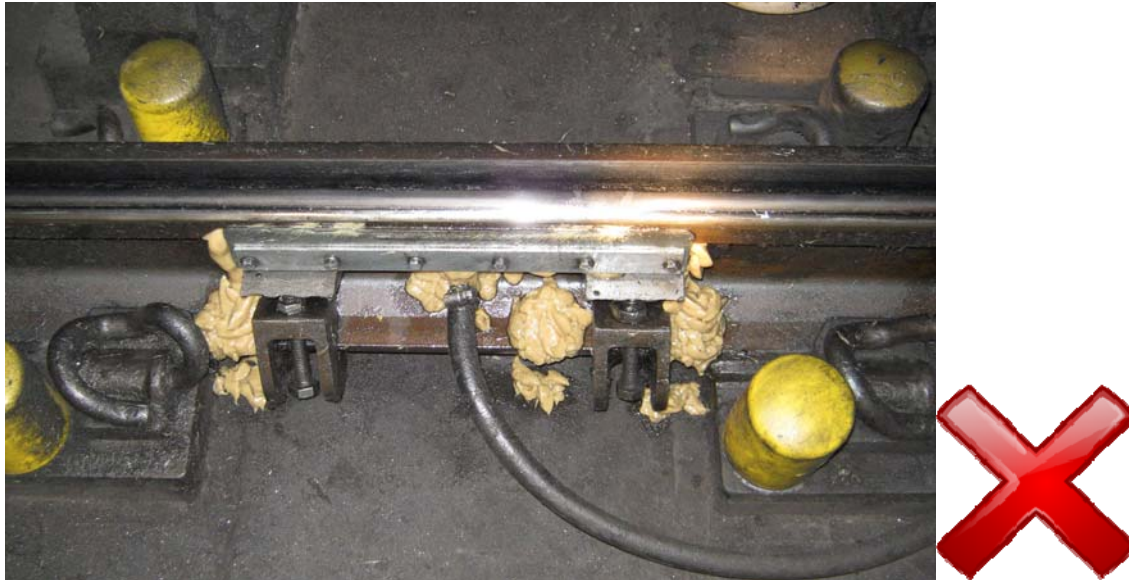
Figure 2 – Lubricator showing leakage of lubricant from the GDU and hose connection. The lubricant is not being transferred to the running edge of the rail. This condition shall be reported as a defect.
