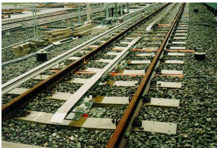
Figure 8 – Low negative shoe detector rail
