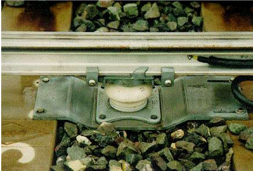
Figure 9 – Low negative shoe detector rail with middle insulator mounted on a special bracket. Note the anchors on either side of the insulator
