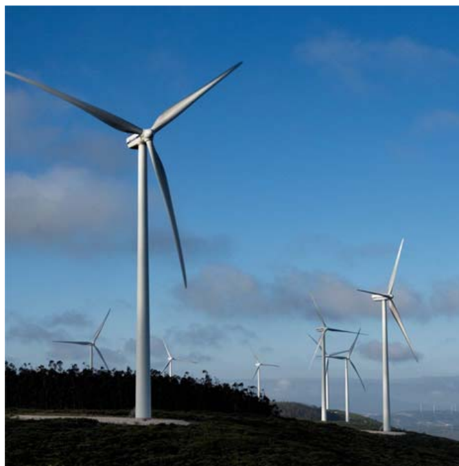
Figure 5 - An Array of 3 MW Vestas Wind Turbines with 90 m Diameter Rotors
