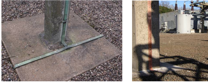
Figure 2 Typical images showing installed stainless steel anchor pin solutions onto concrete structures and equipment foundation pads.
