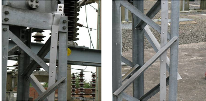
Figure 4 Typical images showing encapsulation of above ground copper tape within capping on a structure that does not lend itself to a direct bolting approach.
