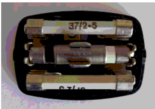
Older Type of Data Link Surge Protection
