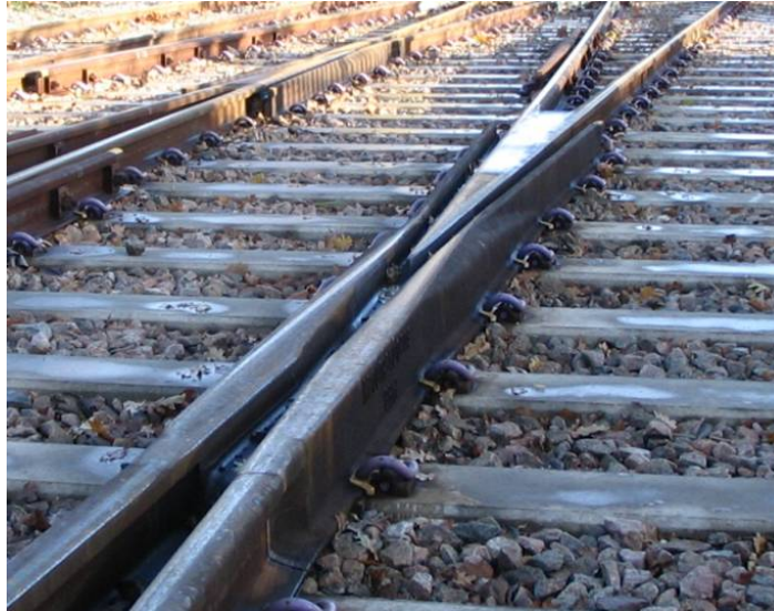
Figure 2 – Welded cast monobloc
