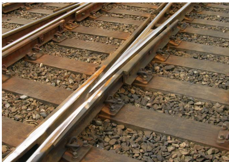
Figure 3 – Cast centre block
