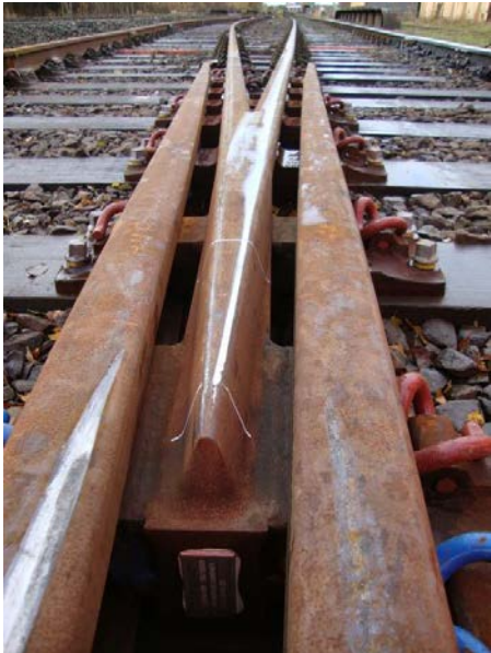
Figure 5 – Machined nose block
