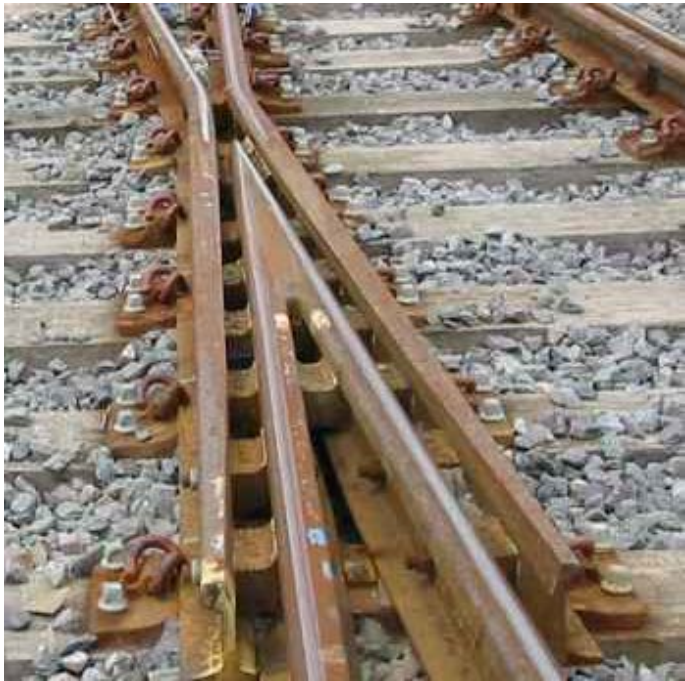
Figure 6 – Electro-slag welded vee
