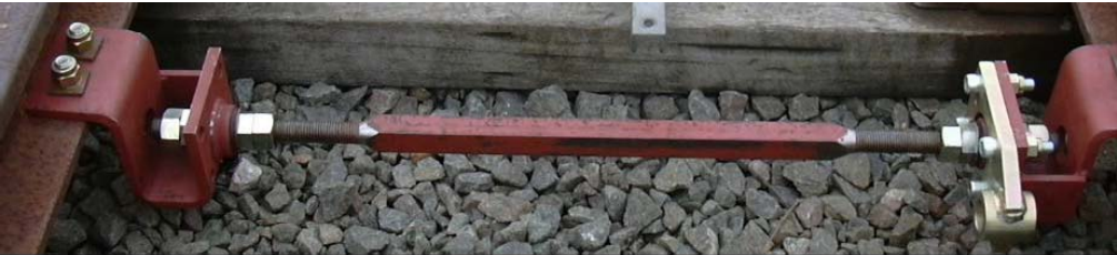
Figure 2 – Adjustable Stretcher Bar Assembly
