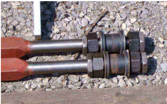
Figure 17 – Full nut/half nut lock nuts
