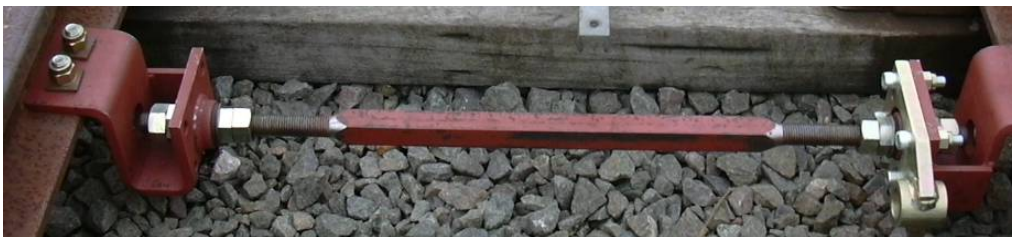
Figure 1 – 35mm adjustable stretcher bar assembly with type 2 brackets
