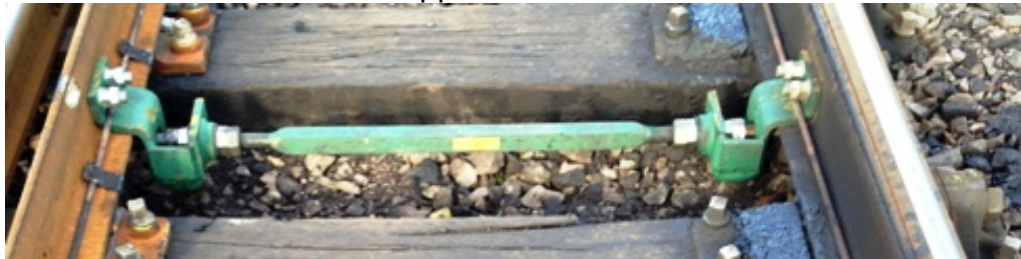
Figure 12 – Full depth 35mm adjustable stretcher bar assembly
