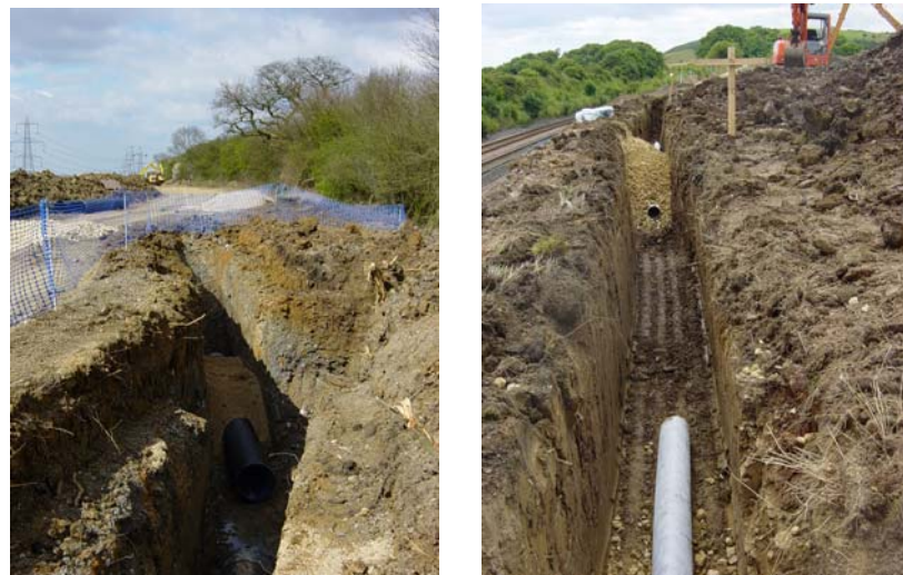
Figure 1E.1: Trench excavation for laying pipes
