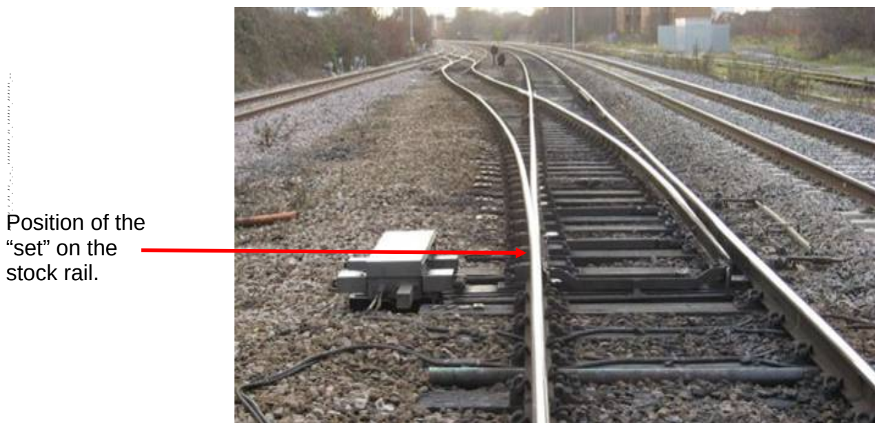
Figure 1 – ‘Set’ of the stock rail
