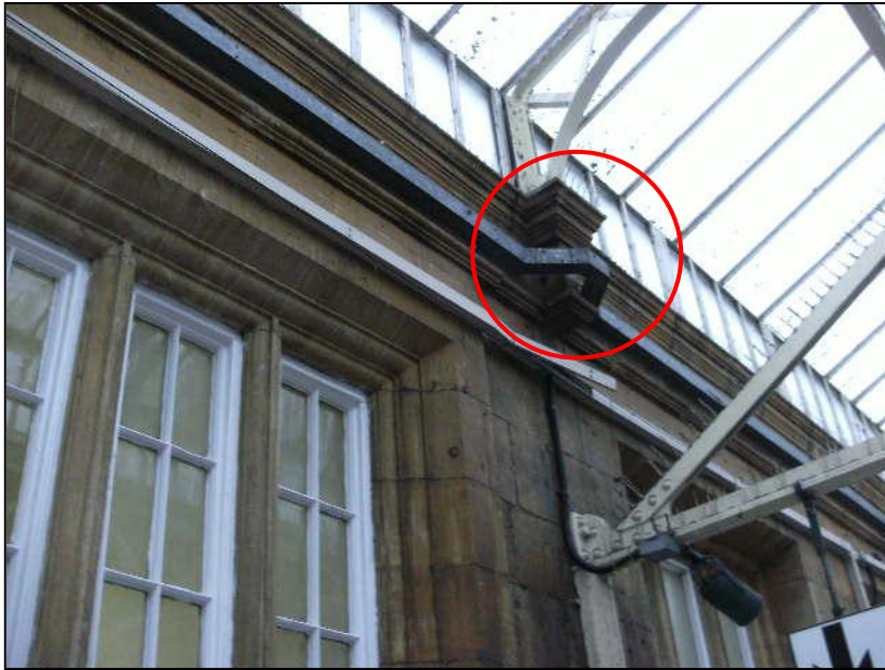
Photograph 2: Showing a typical (intact) section of stone moulding to the same wall
