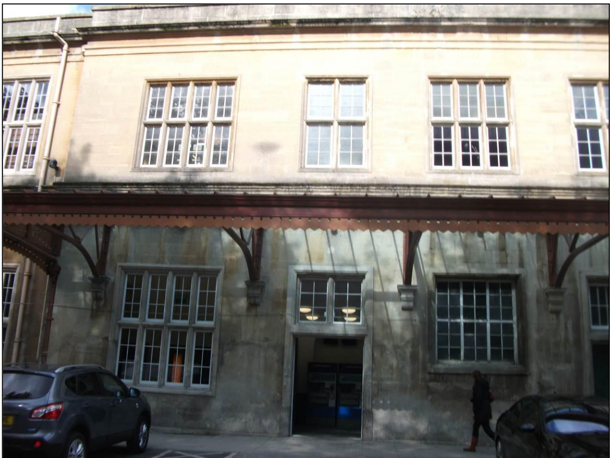
Photograph 3: Bath Spa External Corbel and Parapet Ledge
