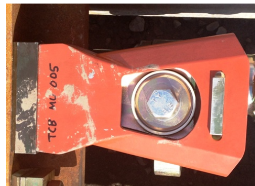
Figure 1 - Web Mounted Motion Units fitted to switch diamonds
