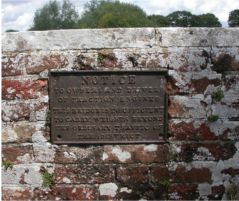
Figure 5 — Fitch's bridge warning sign, UK [11]
