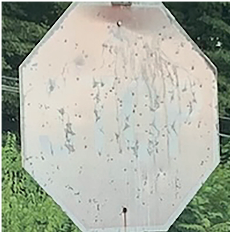
Figure 10 — Faded stop sign
