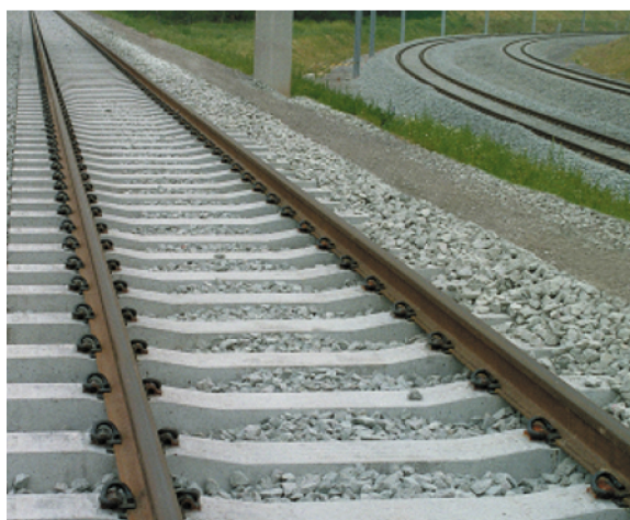
c) Mono-block sleepers
