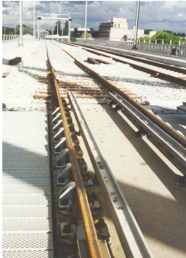
Figure 16 — Special rail expansion device in ballastless track
