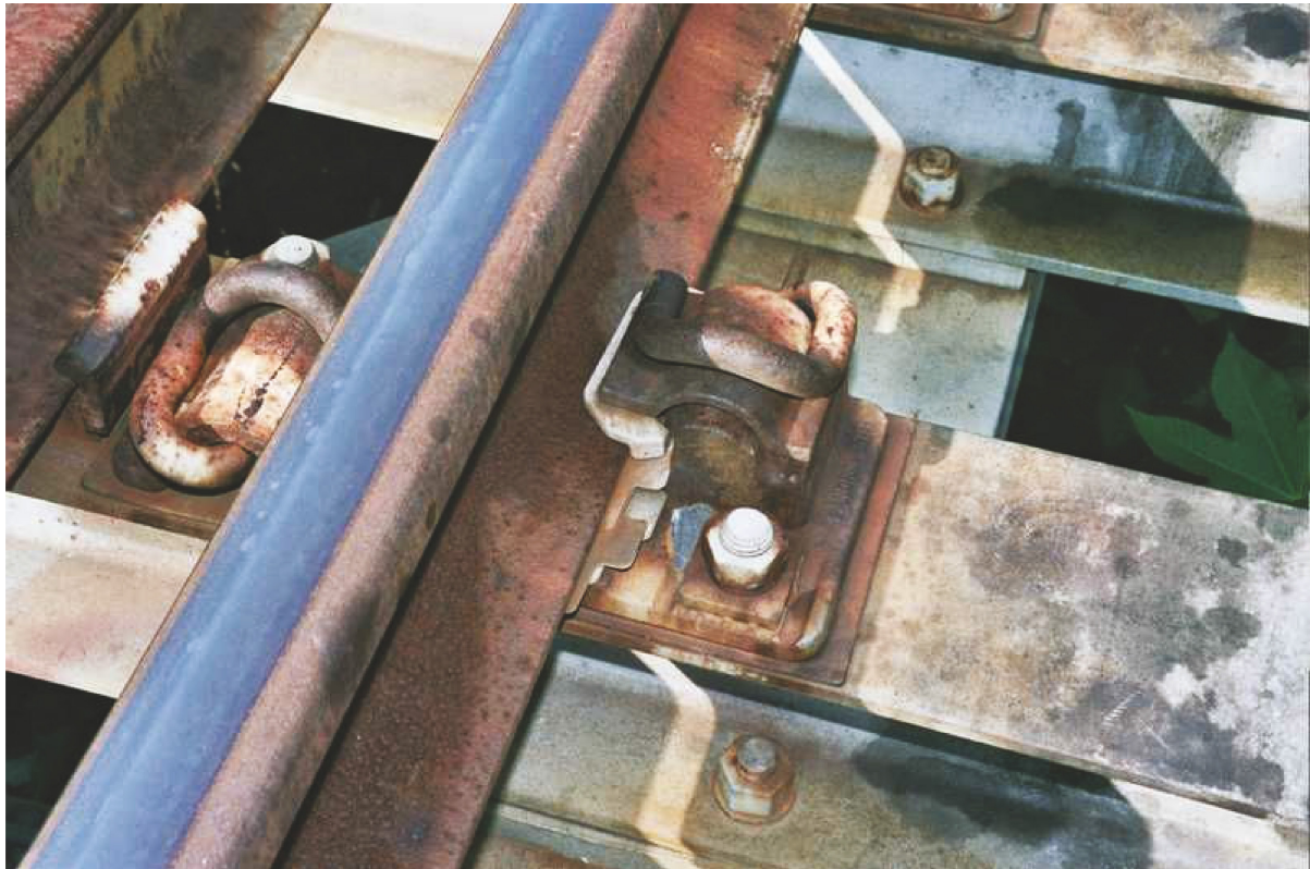
Figure 12 — Zero longitudinal restraint (ZLR) fastening for ballastless track
