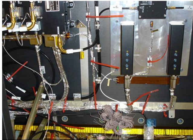
Figure 5-8: Wide strips, fixation by rivets and screws
