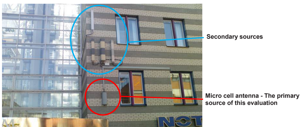
Figure 2.2 Photograph of micro cell antenna
