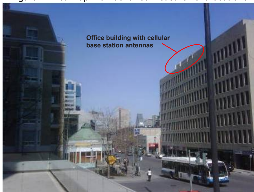
Figure 2: View of the cellular base station antennas from the street
