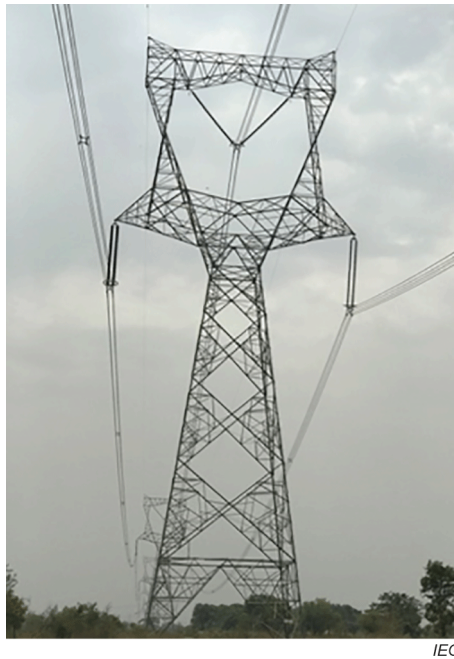
Figure 4 – Typical single circuit delta configuration tower
