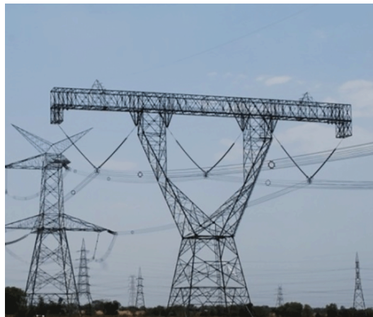
Figure 7 – 1 200 kV single circuit vertical configuration tower
