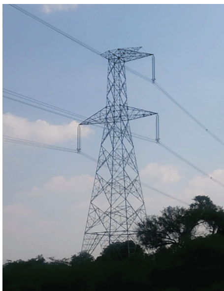
Figure 1 – Typical single circuit vertical configuration tower
