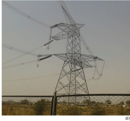
Figure 7 – 1 200 kV single circuit vertical configuration tower
