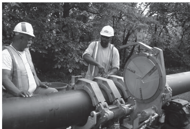
Figure I Joining Large Diameter PE Pipe with Butt Fusion
