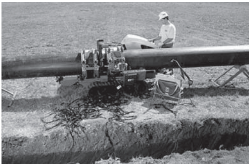
Figure 1 Above Ground Repair with Fusion Machine
