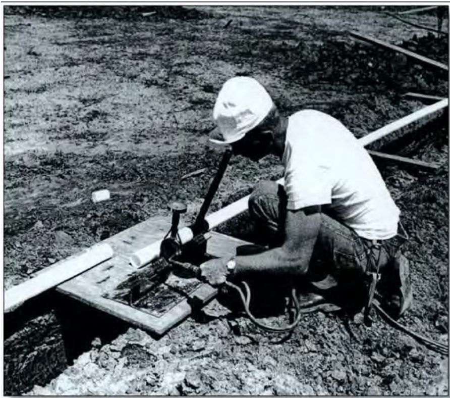
Figure 1: Natural Color Polyethylene Pipe being Fused, 1959, in Caney, Kansas
