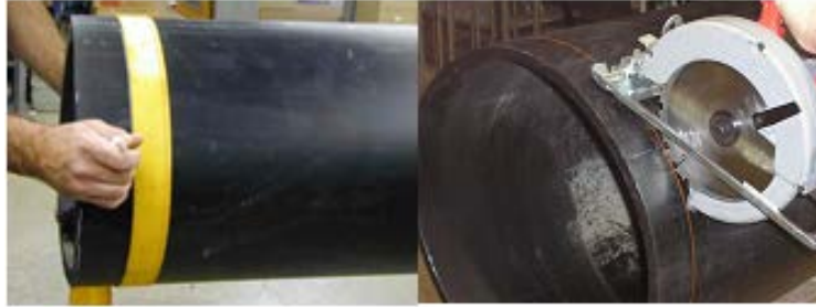
Figure 5: Marking and cutting larger diameter pipes
