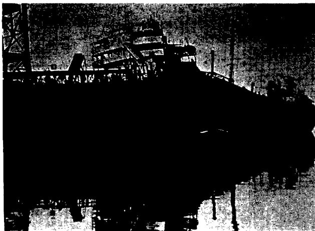
Figure 1. Liberty ship failures from the World War II era: massive hull fractures due to a combination of poor-quality steel, less-than-adequate welding procedures, and low temperatures in the North Sea.
