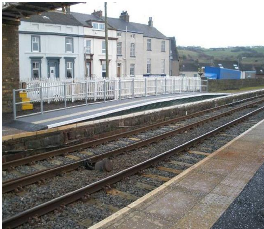
Figure G 1 Harrington Station - example of a localised alteration to achieve standard height platform
